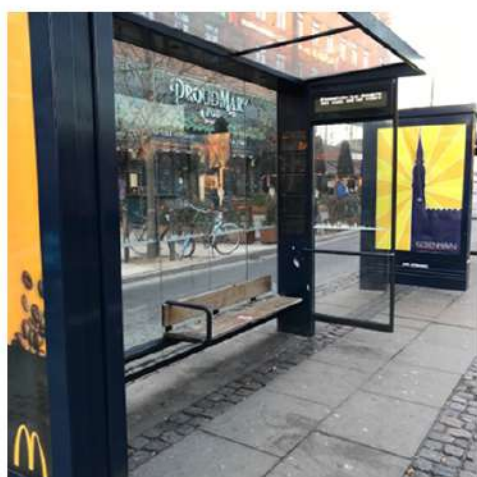
Bus shelter with a small bench and gaps between the glass and the ground.
